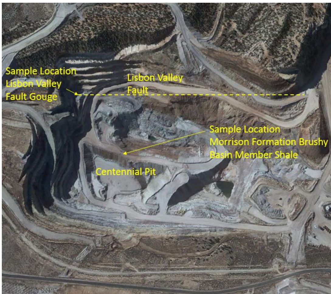
Figure 3.30 Fault Gouge and Morrison Brushy Basin Column Sample Locations
